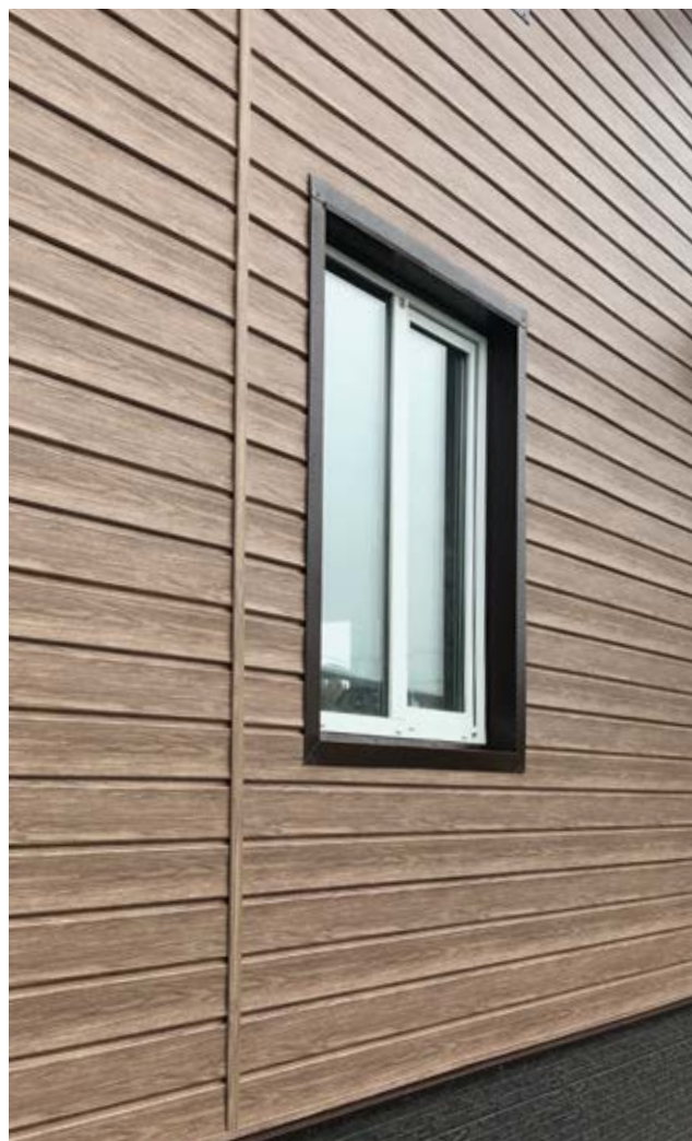
Example of installation of woodgrain LUX series siding
